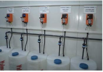
Dosage systems are used for many purposes such as water disinfection,pH reduction and raise, corrosion prevention and so on .
