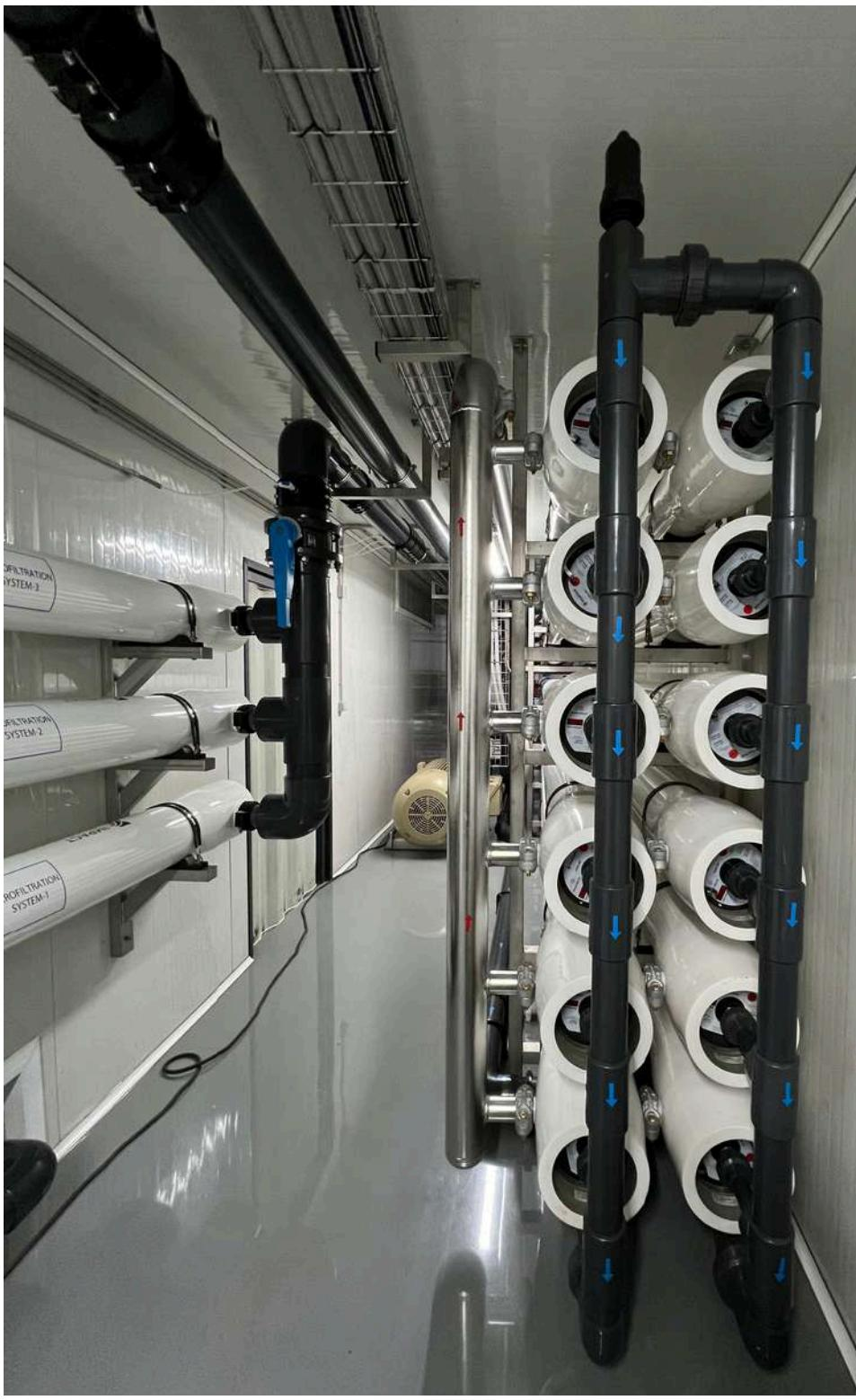
Dissolved organic and inorganic substances (bitter, high conductivity, etc salts, heavy metals, viruses and bacteria in the water are treated with reverse osmosis systems Up to 96 99 of purity in water could be achieved Water with different sources such as well water, tap water, sea water etc could be treated with high purity using Reverse Osmosis Systems.
