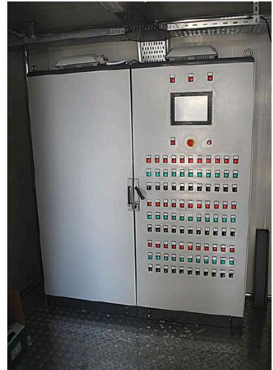
**Electric board, IP 54** is suitable to contain the power, control, monitoring and alarm devices for the plant. The controls shall be identified by metal plates fixed by screws. All instruments shall be safety anchored and located so as to keep proper geometry, both horizontally and vertically.
