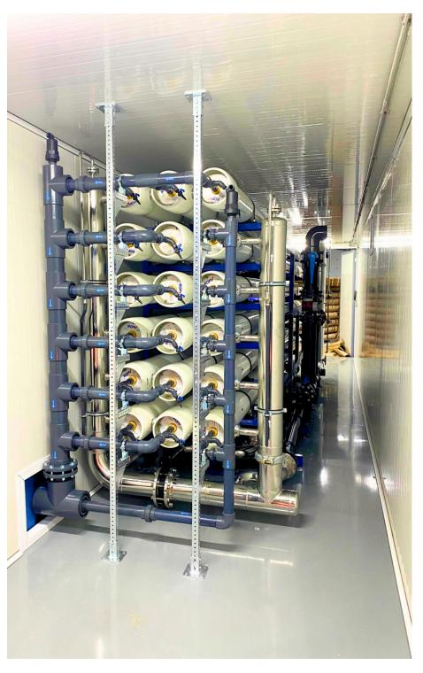
Dissolved organic and inorganic substances (bitter, high conductivity, etc salts, heavy metals, viruses and bacteria in the water are treated with reverse osmosis systems Up to 96 99 of purity in water could be achieved Water with different sources such as well water, tap water, sea water etc could be treated with high purity using Reverse Osmosis Systems.
