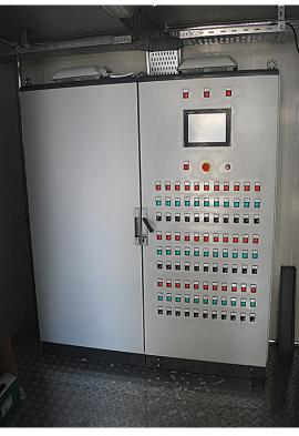
Electric board, IP 54 is suitable to contain the power, control, monitoring and alarm devices for the plant. The controls shall be identified by metal plates fixed by screws. All instruments shall be safety anchored and located so as to keep proper geometry, both horizontally and vertically.
