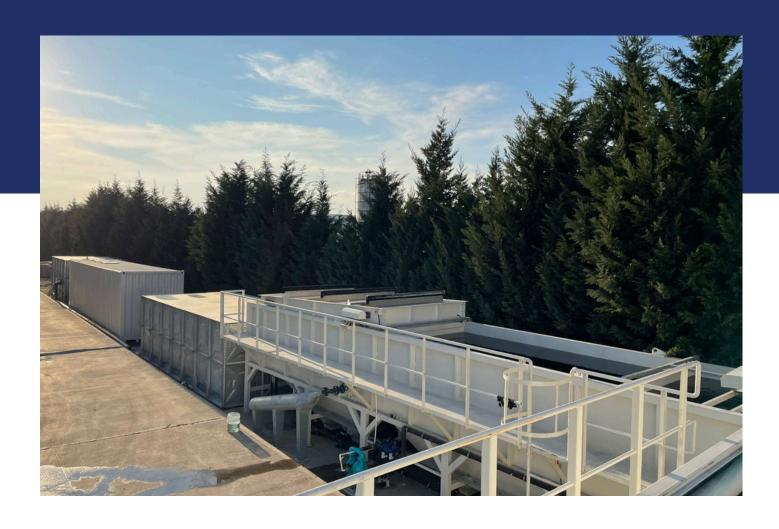
The textile wastewater recovery system has the capacity to treat 90% or more of the wastewater from the textile washing and dyeing industry, thus contributing to the company's economy. You can use the textile wastewater recovery system without the need for a separate building and an additional area. In the textile waste water recovery system the system is prepared and delivered in a container. At the same time, you can easily increase the capacity by placing additional container.
